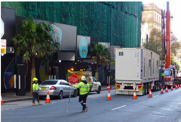
Figure 8: Through traffic lane/s adjoining a work area must be supervised by authorised traffic controllers.
