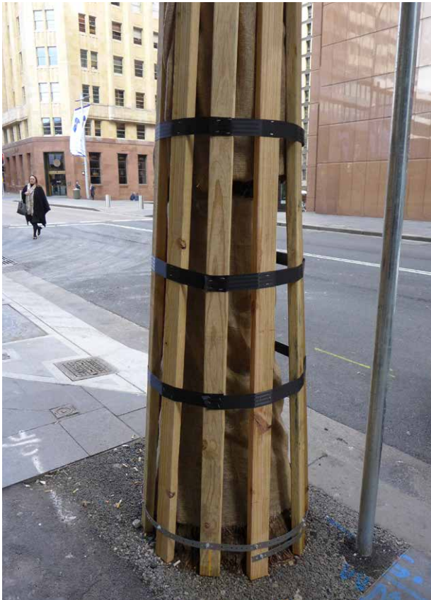
Figure 33: Typical required tree trunk protection.
