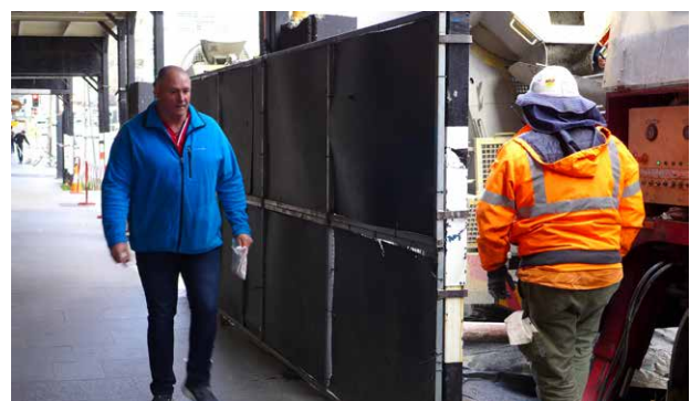
Figure 19: The use of screens to protect pedestrians and bicycle riders at concrete pumping locations is generally not supported by the City . Where however approval is given temporary screens must be of a durable quality, satisfactory design and fixed securely in place when in use. Screens must be removed from the public place immediately following completion of daily pumping operations.
