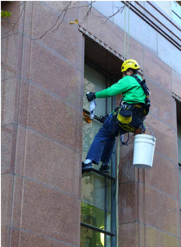
Figure 26: Rope access ( hoisting activity) to undertake minor maintenance activity e.g.: window cleaning, is permitted subject to approval being given to establish exclusion zones (see Figure 25 ) based on risk assessment by the PCBU and implementing any necessary control measures . All ropes are to be contained within the pedestrian exclusion zone.
