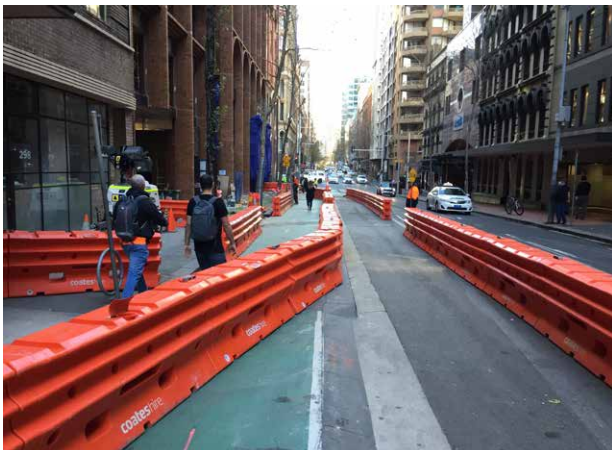
Figure 16: Temporary pedestrian and bicycle rider diversions should be avoided. Where works are proposed that require temporary closure of footways / cycleways , the City may agree to temporary diversions being established subject to meeting minimum design standards.
