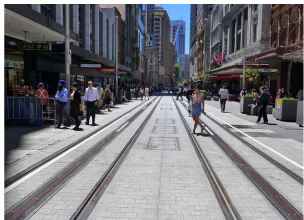
Figure 1: Restrictions apply when working within and adjoining a light rail corridor. Proponents must make themselves aware of the light rail operator's requirements when planning works.
