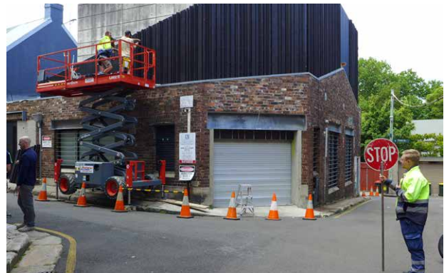
Figure 10: Where approval is given to establish and operate hoisting devices on roadways , special controls will generally need to be implemented including traffic / pedestrian control measures.
