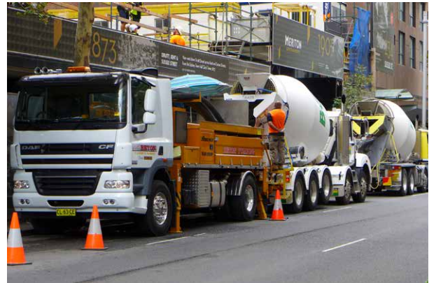
Figure 29: To minimise impacts on the local road network and pedestrian / bicycle rider movement, work zones must be appropriately managed and operate at all times in accordance with the conditions of approval including directions of authorised persons . See also 4.4.2 in relation to the use of footway / kerbside barriers in works zones .
