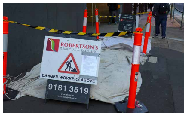
Figure 25: Exclusion zones required by the PCBU beneath rope access hoisting activity must be of adequate stability, visibility and positioned to minimise footway obstruction. For some activities drop-sheets to protect the footway surface may be necessary or required. Where used, sheets must be placed wholly with the exclusion zone/s to eliminate pedestrian trip hazards.
