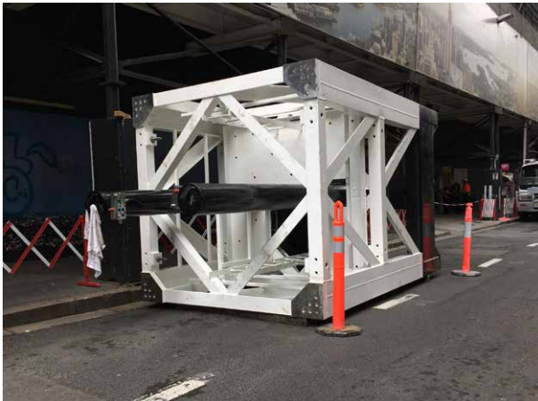
Figure 31: Works zones are granted for the primary purpose of standing vehicles to load and unload. They must not be used for other purposes such as the storage of equipment or material unless otherwise specifically approved.
