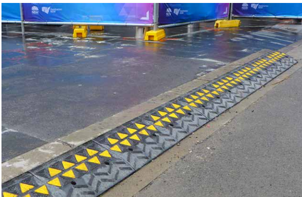
Figure 9: Temporary rubber-type ramps must be used to allow small vehicle access to approved works on footways . Note: This form of access may not be suitable where older fragile sandstone kerbing is present or where access by large heavy vehicles / equipment such as forklifts and scissor lifts are to be used. Contact the Construction Regulation team for further advice and direction.
