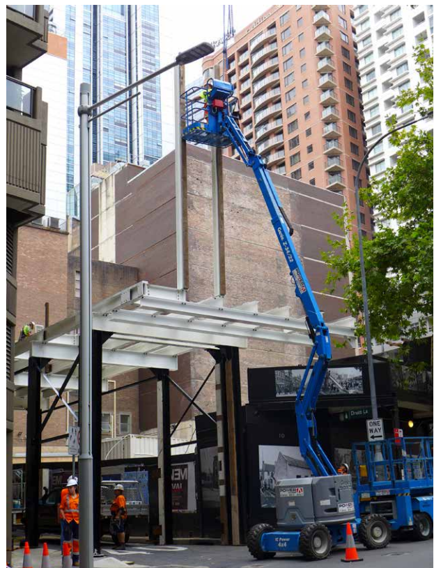
Figure 12: Hoist installations on hoarding decks are only permitted under special circumstances. Where approved , parked hoist cars at deck level must be fully screened by hoarding fascias including on the sides. Any mesh used to screen the hoist structure must meet the minimum flammability performance criteria in the City's 'Guidelines for Hoardings and Scaffolding'.
