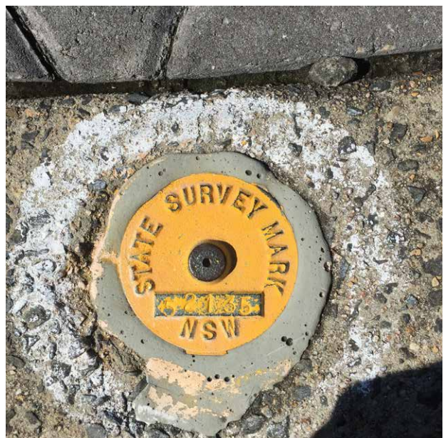
Figure 46: Examples of survey marks located in the City of Sydney LGA. Survey marks are important survey assets and are protected under legislation.
