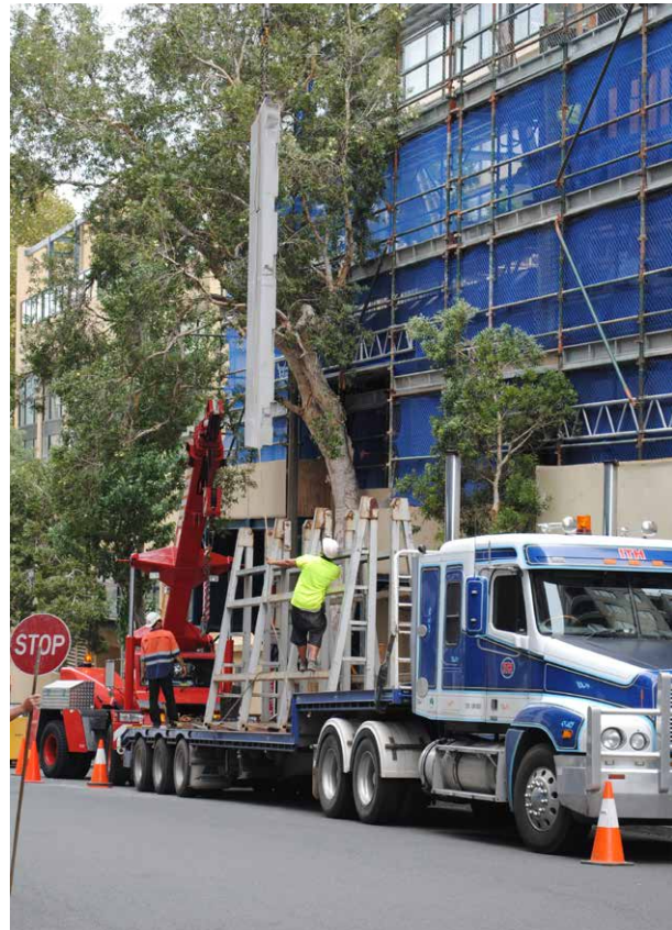
Figure 32: Appropriate site management practices must be fully implemented and followed to prevent damage to street trees when undertaking hoisting activities.
