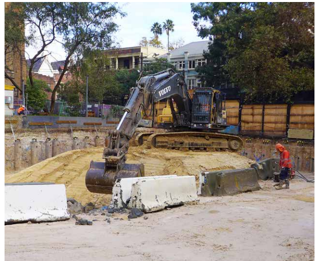
Figure 45: The short-term stockpiling of excavated material that is awaiting removal from a site is permissible subject to specific approval and implementing environmental controls including measures to prevent the movement of material in water run-off and through wind actions.
