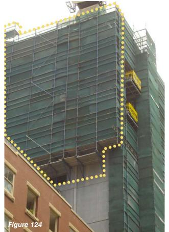
**Note (1):** In proposing a *cantilevered work platform* it is the responsibility of the person undertaking the work to satisfy the relevant provisions of the Work Health and Safety Act 2011 and Regulations in relation to public safety below a work area.
