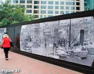
fascias must be covered by a graphic display (which also includes any proposed signage as set out in Table 2) with the remaining surface finished and painted flat black or other approved colour appropriate for the graphic display. For Type B highbay hoardings where the deck height is greater than 3 metres the graphics must be installed on the site fence up to at least the lateral bracing elements.
