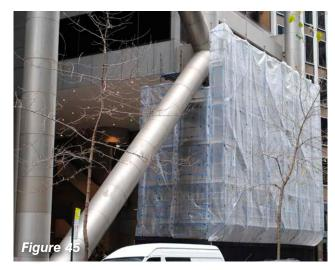
**Figure 43:** Screening of scaffolding using a high-quality scaffolding wrap is particularly appropriate in prominent locations and on historic buildings.
