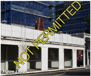
**Figures 27(a), (b) and (c):** These three forms of temporary structures and installation are NOT PERMITTED on footways and roadways within the City of Sydney area.
