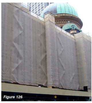
**Figure 125:** Temporary structures must not encroach on frontages of adjoining properties unless specifically approved by the *City*.
